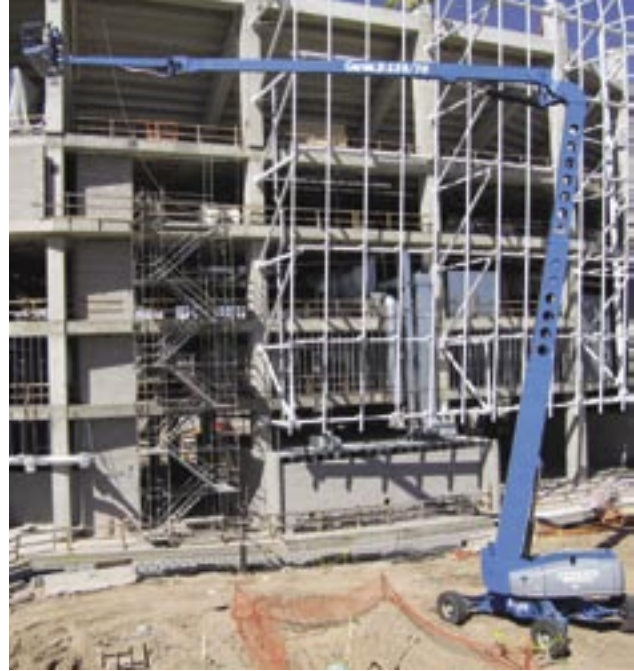
An OPTCO crew member touches up stadium steel at nearly 120 ft.
