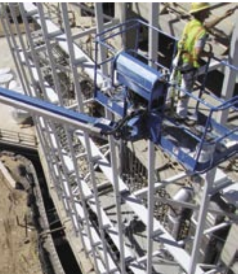
The Genie Z-135/70's ability to quickly articulate vastly improved touch-up production.
